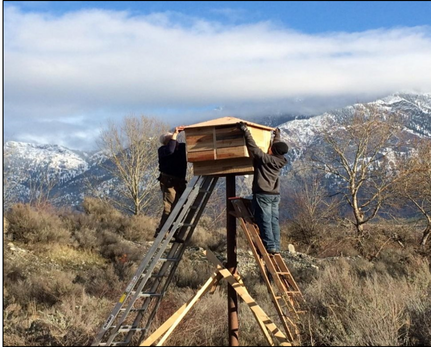
Figure 14. A mini condo is installed in late fall at Lillooet, British Columbia. Photo contributed by V. Birch-Jones. This structure is larger and offers more roost microclimate options than a standard multichambered bat box. This particular design was modified to contain a pillar of sand in the middle to function as a heat sink – stable and warm at night for pups, but unlikely to overheat despite the fact that this region is typically the hottest location in Canada (outdoor ambient temperatures have reached 47°C or 117°F; Environment Canada 2021). This site will continue to be monitored for effectiveness.
